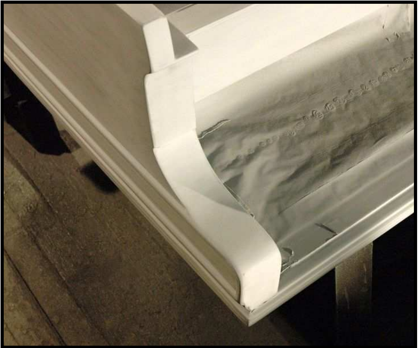
Detail after primer coats, of repaired area.
